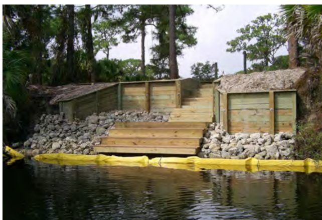
Original 2005 constructed structure
