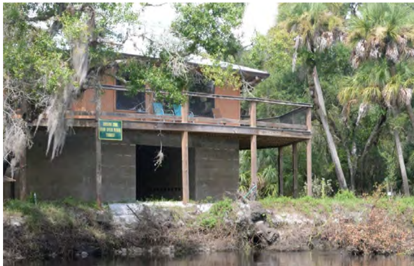
Pre-construction project area.
